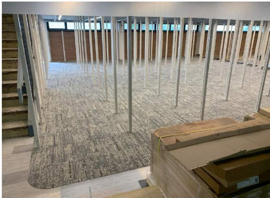
Installed flooring throughout basement and 1<sup>st</sup> Floor (protected) and support columns under mezz painted
