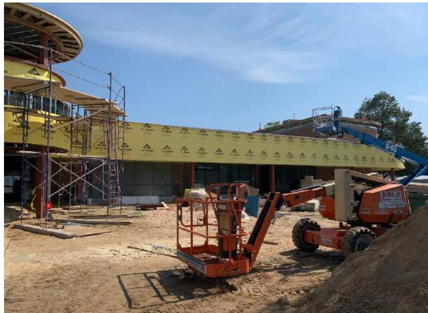
Rotunda and North soffit sheathed with densglas
