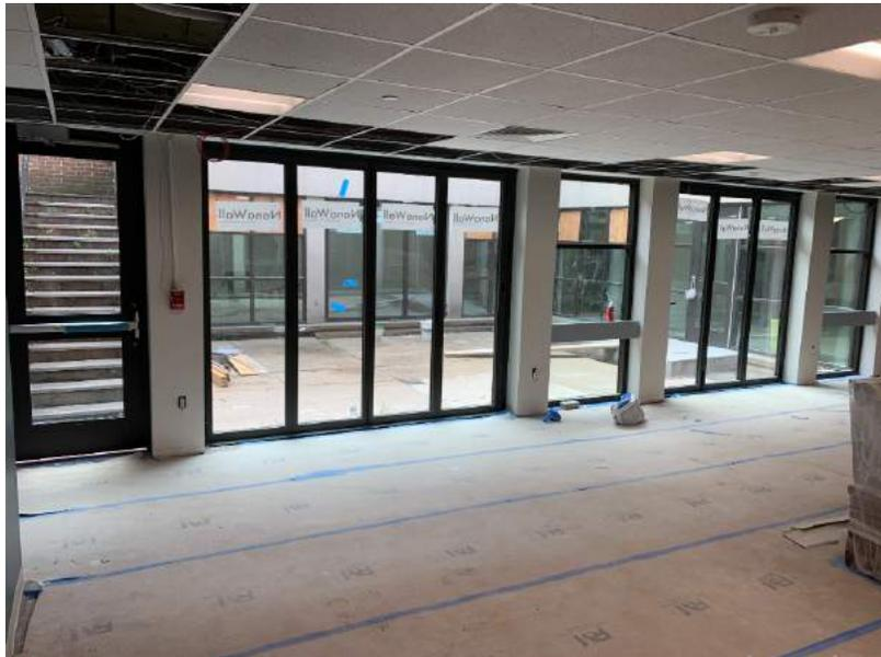
Axiom trim installed and ceiling whited out. All basement courtyard windows installed.
